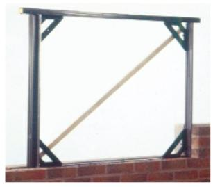
Strong reusable profile brackets allow *Kingspan* **Therma**bate® to be used as an alternative to temporary timber templates for forming openings in walls where frames are fitted at a later stage.
