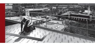
Xtratherm FR/TP Thermal Ply is a composite insulated panel of Xtratherm Polyisocyanurate core with a composite foil face, bonded to 6mm WBP grade plywood. FR/TP is designed to provide high levels of thermal insulation and decking in one operation for new and refurbishment flat roof applications.
