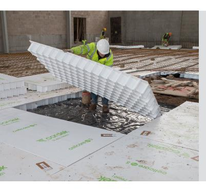
The Cellcore HX range of collapsible products have been designed to protect foundations from the effects of ground heave.
