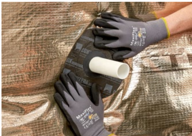
Fix grommet around pipes and ducting
