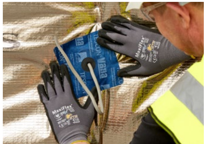
Fix grommet around electric wiring
