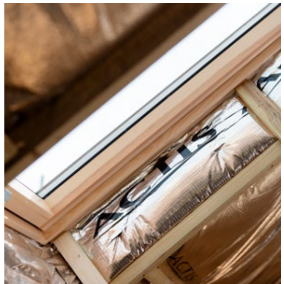
Perimeter edges: Stapled, taped, secured with batten
