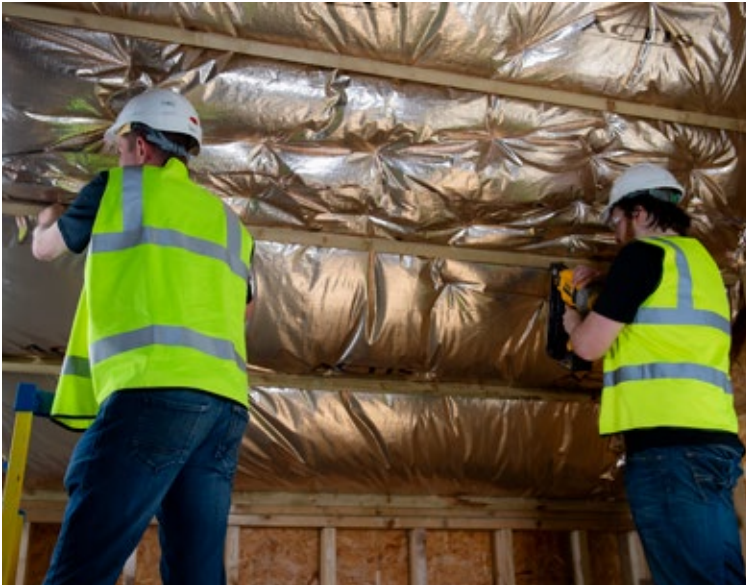
Prepare for plasterboard fixing
