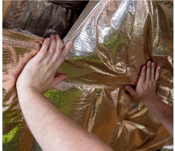
Seal with integral tape
