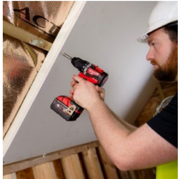
Fix plasterboard
