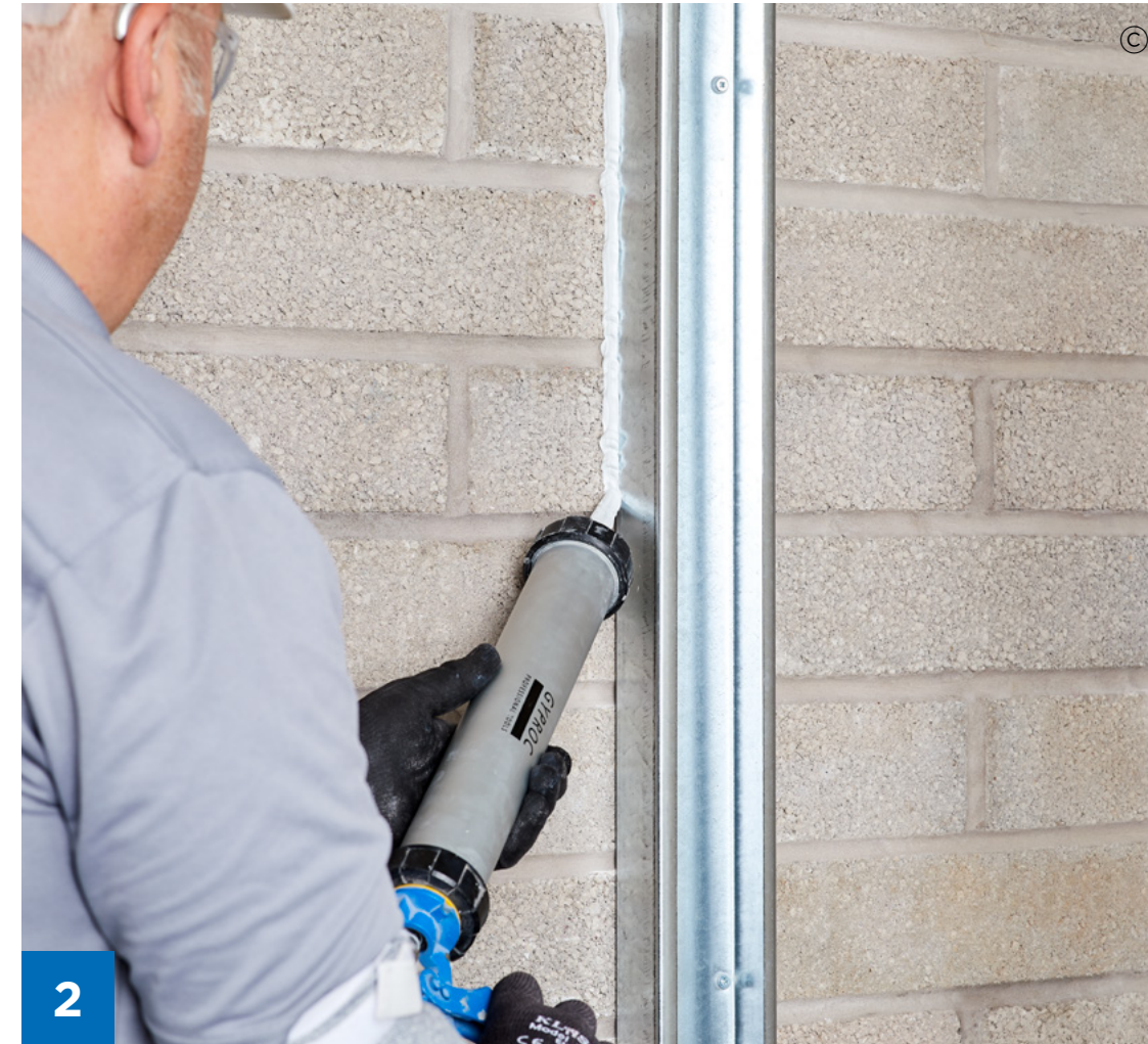
Before offering any boards into position, a continuous 6 mm wide bead of Glasroc X Sealant is needed along the vertical edge of the surface that the first sheet of Glasroc X Sheathing Board will abut.
