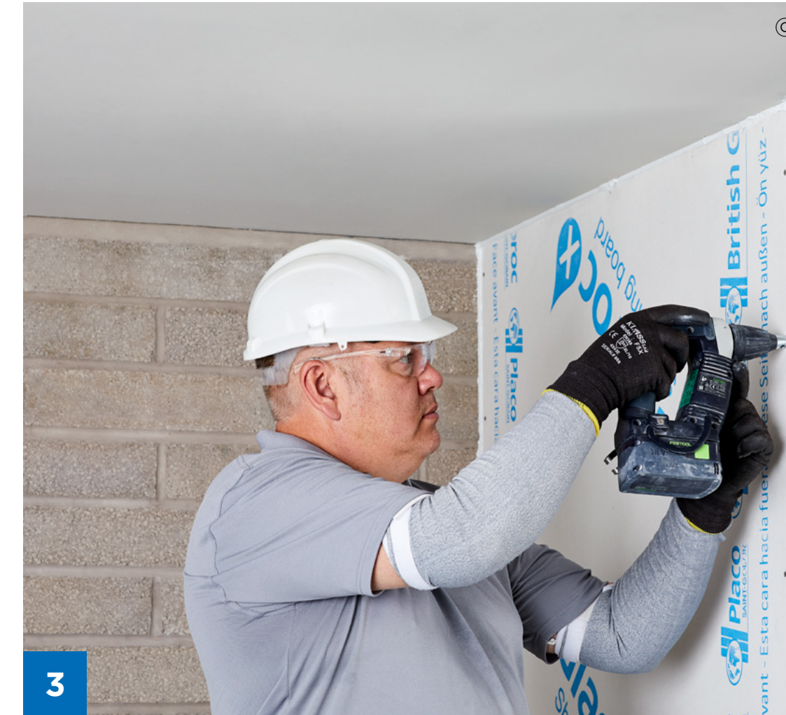
Use Glasroc X Screws 25 mm to fix Glasroc X Sheathing Board to the SFS framework.
