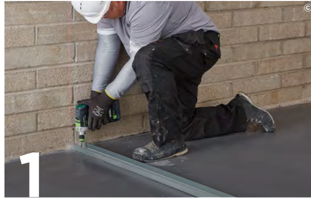
1 Suitably fix the appropriate Gypframe Floor & Ceiling Channels to the floor and soffit at the required centres.
