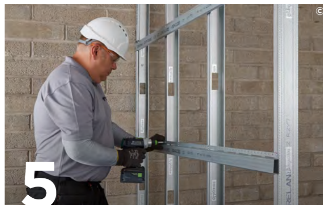
5 Transverse fix Gypframe RB1 Resilient Bars to the stud framing. Join Gypframe RB1 Resilient Bars by nesting them together over a Gypframe 'C' Stud using British Gypsum Wafer Head Drywall Screws.
