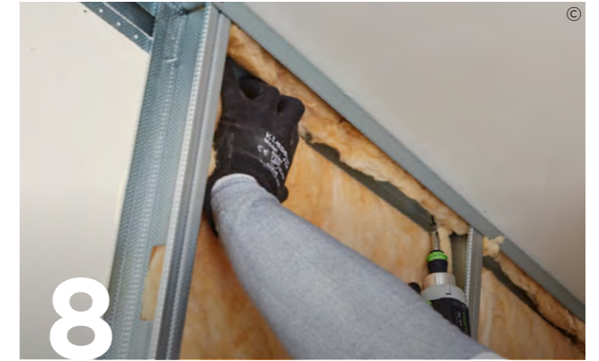
8 Add Isover Acoustic Partition Roll (APR 1200) insulation to the partition cavity for optimal acoustic performance.
