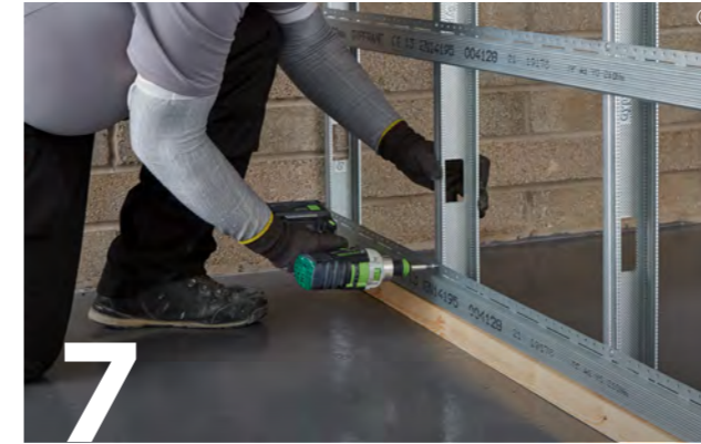
7 Where Gypframe RB1 Resilient Bars are fixed transverse at the lowest point on the partition, a timber nogging should be suitably fixed beneath the Gypframe RB1 Resilient Bars to stop it being trapped when skirting is installed.
