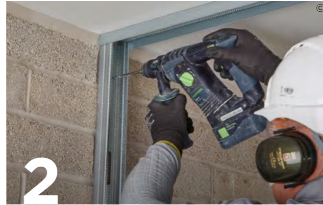
2 Fix Gypframe 'C' Studs to abutments and openings using suitable fixings.
