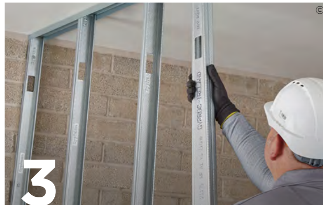
3 Friction fit Gypframe 'C' studs into the appropriate Gypframe Channels at required centres.
