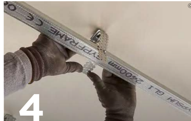
4 Bend the protruding legs of each bracket to sit back from the channel face.
