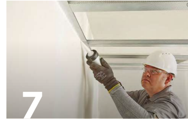
7 Use Gyproc Sealant to seal the perimeter of each frame.
