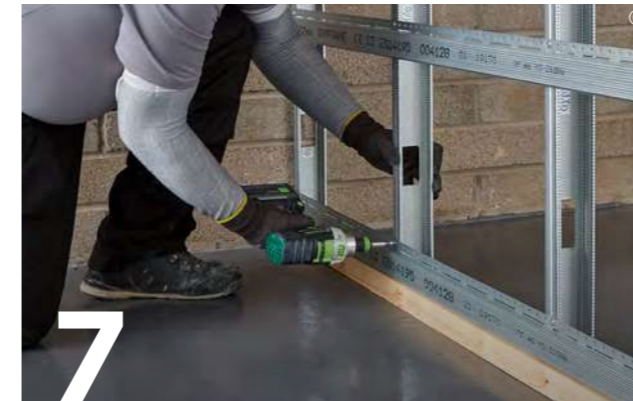
Where Gypframe RB1 Resilient Bars are fixed transverse at the lowest point on the partition, a timber nogging should be suitably fixed beneath the Gypframe RB1 Resilient Bars to stop it being trapped when skirting is installed.
