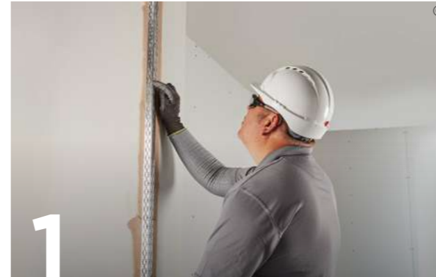
1 A Thistle Thin Coat Angle Bead is fixed to the plasterboard angle by embedding in dabs of finish plaster.
