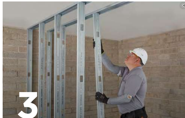
3 Friction fit Gypframe 92 S 10 'C' Studs into the appropriate Gypframe Channels at the required centres.
