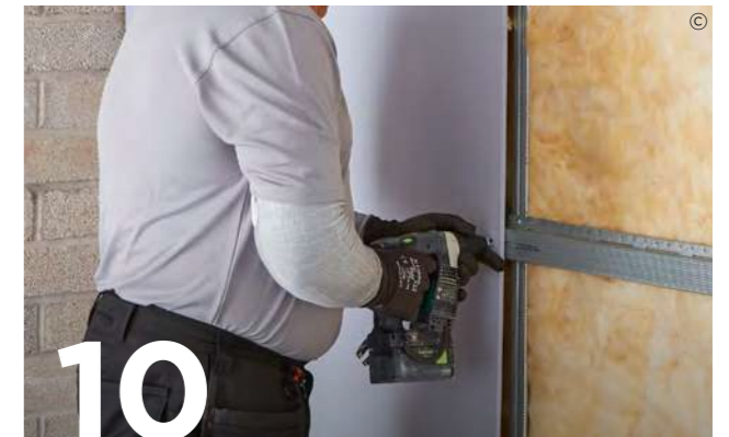
Use British Gypsum Drywall Screws to fix Gyproc plasterboards to the Gypframe RB1 Resilient Bars, with all joints staggered.
