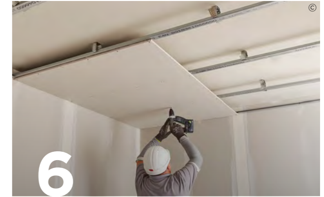
6 Suitably fix boards to form one or two layer linings as specified using appropriate fixing at 90 degrees to the Gypframe GL1 Lining Channels and Gypframe GL8 track.
