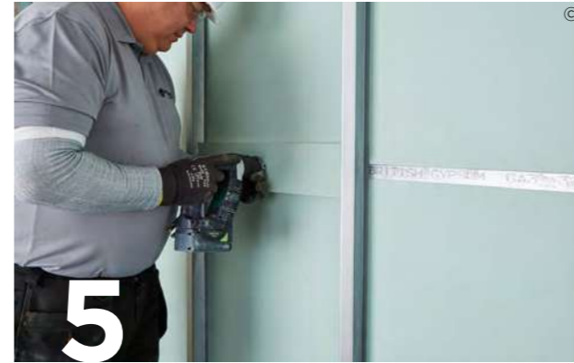
5 Fire stop horizontal board joints using Gypframe GA3 Angle and strips of Gyproc CoreBoard from the non-shaft side.
