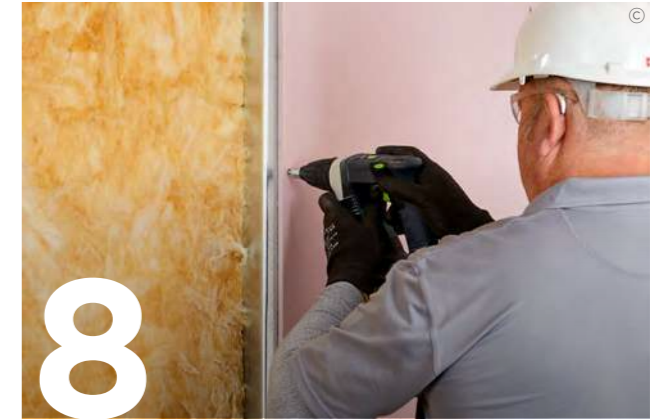
8 Use British Gypsum Jackpoint Drywall Screws to fix Gyproc plasterboards or Glasroc specialist boards to the SFS framework.
