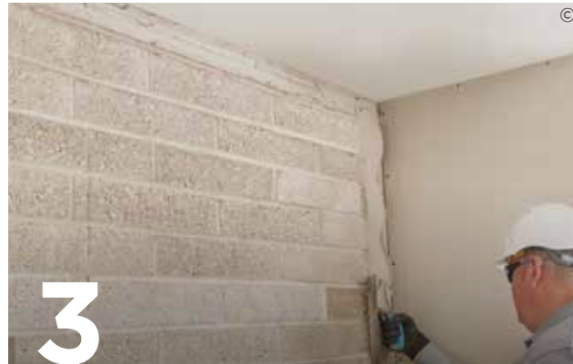
3 When fixing directly to masonry backgrounds Gyproc DriWall Adhesive is applied in a continuous ribbon to the wall perimeter and around all services and openings. This is particularly important if the lining is designed to act as an air barrier to achieve building airtightness.
