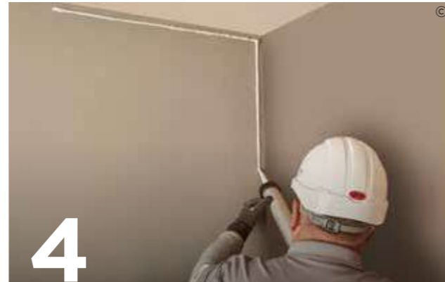
4 When fixing directly to plastered masonry backgrounds Gyproc Sealant is applied in a continuous fillet/ribbon to the wall perimeter and around all services and openings. This is particularly important if the lining is designed to act as an air barrier to achieve building airtightness.
