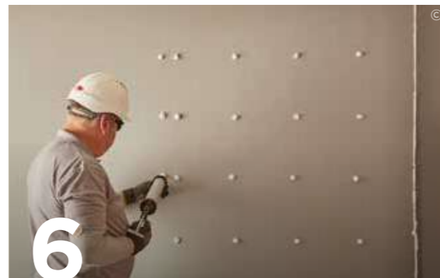
6 If using Gyproc Sealant, gun-apply to the wall, in blobs at 300 mm centres.
