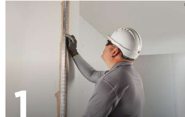
1 A Thistle Thin Coat Angle Bead is fixed to the plasterboard angle by embedding in dabs of finish plaster.
