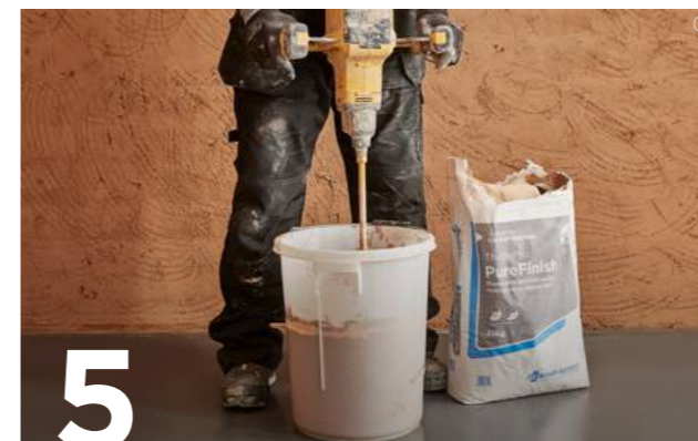
5 Mix Thistle plasters by adding to clean water and using clean mixing equipment. Avoid contamination from previous mixes as this can adversely affect the setting time and strength.
