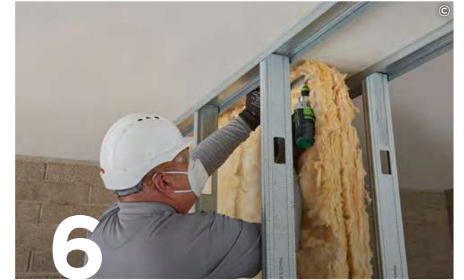
6 Add Isover Cladding Roll 40 insulation to the partition cavity for optimal acoustic and thermal performance.
