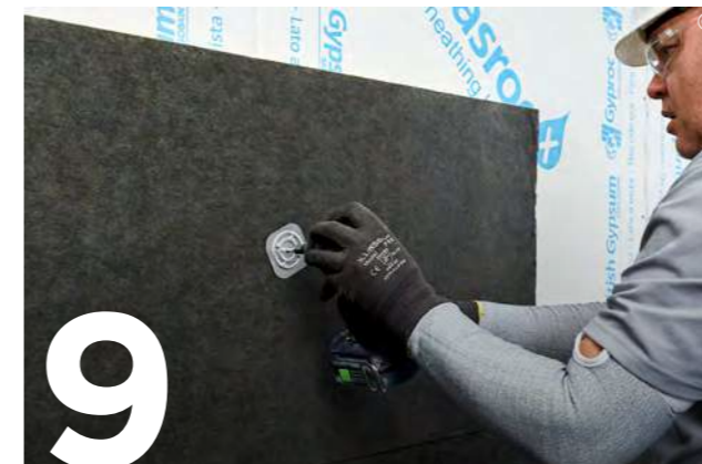
9 Isover Polterm Max Plus to be fixed through the Glasroc X Sheathing Board into the SFS framework.
