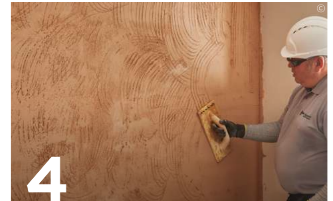
4 Rule the final coat to an even surface and lightly scratch to form a key.
