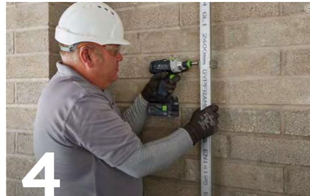
4 Bend Gypframe GL2 or GL9 Bracket leg forward. Use British Gypsum Wafer Head Drywall Screws to fix each leg to the Gypframe GL1 Lining Channel.
