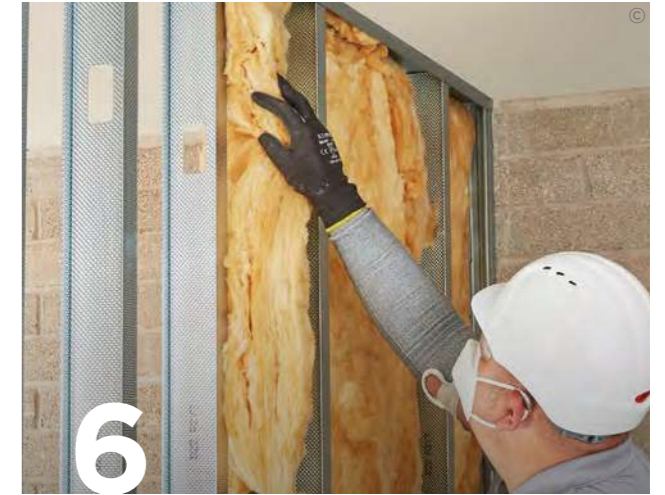
Add Isover Acoustic Partition Roll (APR 1200) insulation to the partition cavity for optimal acoustic and thermal performance.
