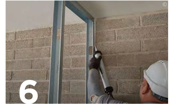
6 Use Gyproc Sealant to seal the perimeter of the partition.
