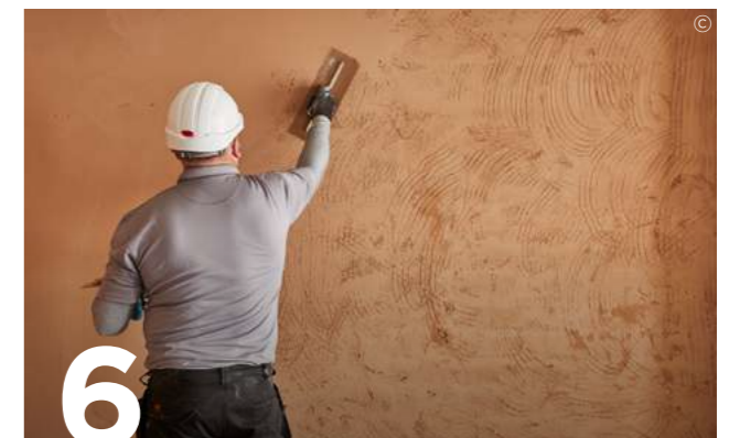
6 Allow the Thistle Undercoat Plaster to set. Apply Thistle Finish Plaster with firm pressure, build out to the required thickness in two applications and trowel to a smooth matt finish. It may be necessary to control the suction with Thistle GypPrime. Good site practice should be followed, as outlined in BS EN 13914-2. Design considerations and essential principles for internal plastering.
