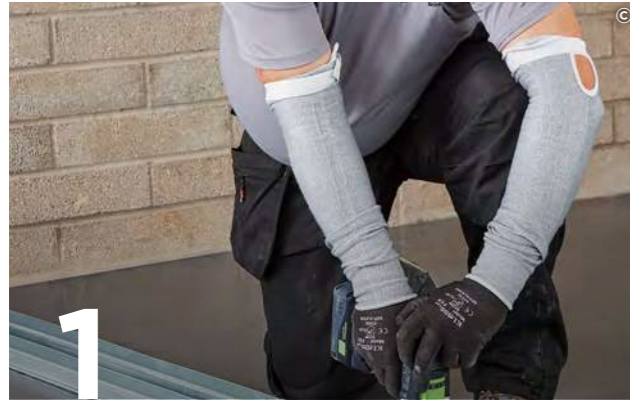
Suitably fix the appropriate Gypframe Floor & Ceiling Channels in two rows at the required centres to the floor and soffit.
