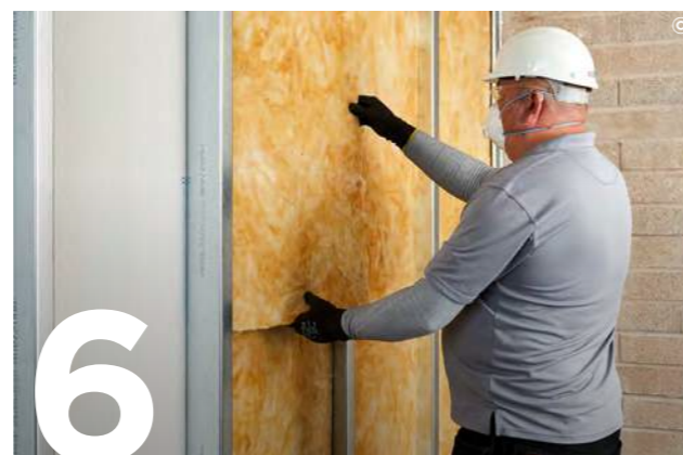
6 Add appropriate Isover insulation within the cavity.
