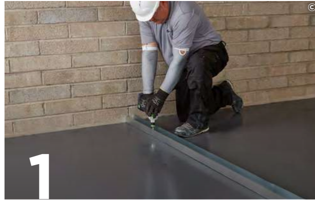
1 Suitably fix the appropriate Gypframe Floor & Ceiling Channels at the required centres to the floor and soffit.
