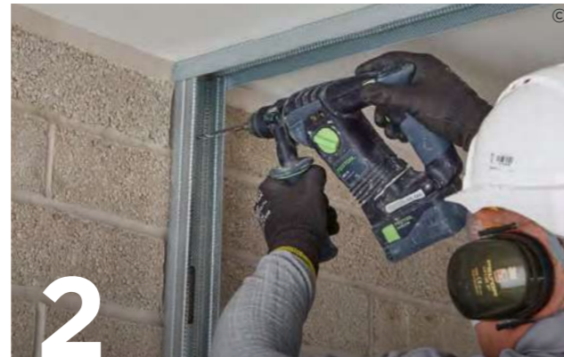
Fix Gypframe 'C' Studs to abutments and openings using suitable fixings.
