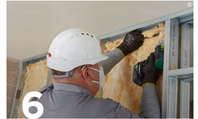
Add insulation to the partition cavity for optimal acoustic and thermal performance.
