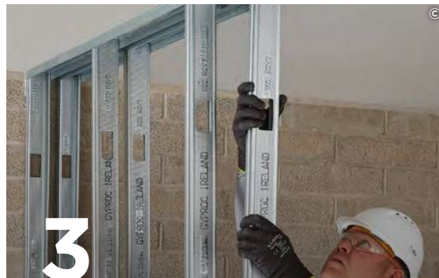
Friction fit Gypframe 'C' Studs into the appropriate Gypframe Floor & Ceiling Channels at the required centres.
