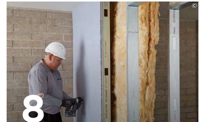
8 Use British Gypsum Jack-Point Screws to fix Gyproc plasterboards to the Gypframe framework.
