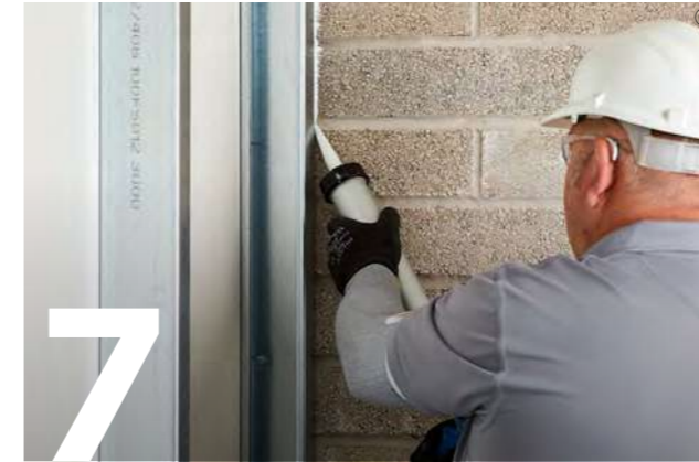
7 Use Gyproc Sealant to seal the perimeter.
