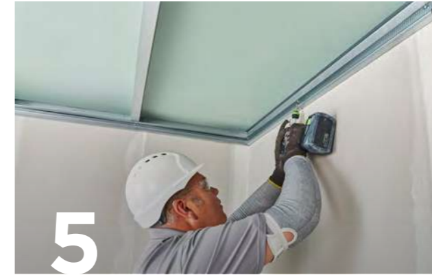
5 Fix the Gypframe MF6 Perimeter Channel directly to the starter channel and floor and ceiling channels using appropriate fixings.
