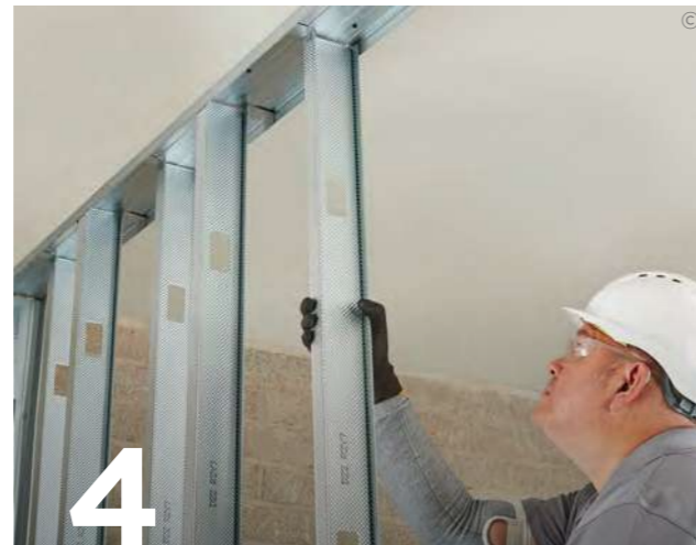
Friction fit Gypframe 'I' Studs into the Gypframe Floor & Ceiling Channels. Alternating the direction of the clip at the top and bottom of the stud to create a staggered stud framework.
