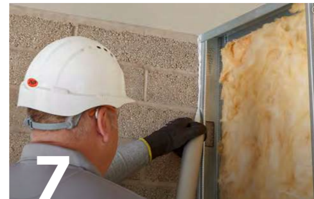
Use Gyproc Sealant to seal the perimeter of the partition.
