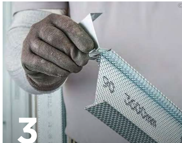
Insert Gypframe Spacer Clips to the top and bottom of the studs. Use Gypframe SC1 when using Gypframe 60 | 70 'I' Studs. Use Gypframe SC2 Spacer Clips when using Gypframe 92 | 90 'I' Studs.
