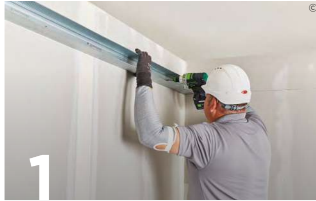
1 Suitably fix the appropriate Gypframe floor and ceiling channels to the perimeter at the required centres. Channels are located along the perimeter that will receive the 'I' Studs.
