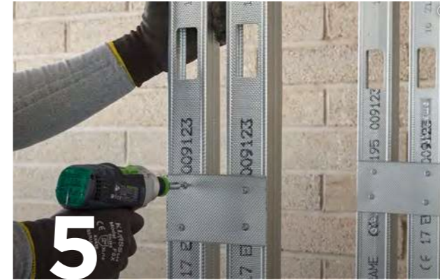
Brace the two frameworks with a Gypframe 99 FC 50 Fixing Channel attached to the Gypframe 'C' Studs at 1200 centres. Use two British Gypsum Wafer Head Drywall Screws per junction.
