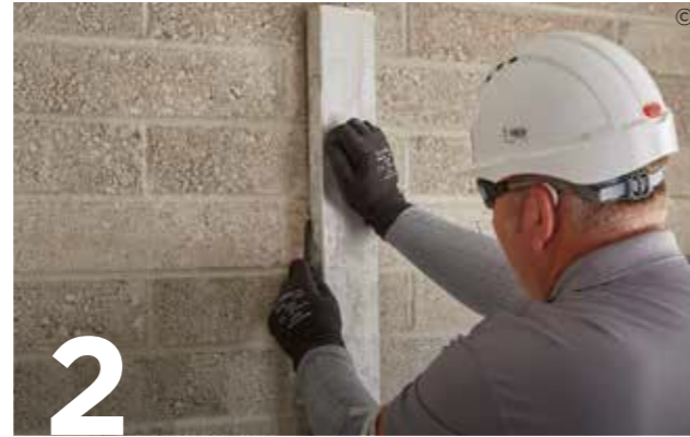
2 Mark the board edge positions on the wall or plasterboard to aid the correct and accurate application of the chosen DriLyner Dab system.
