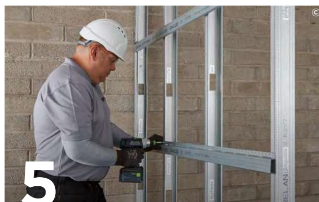
Transverse fix Gypframe RB1 Resilient Bars to the stud framing. Join Gypframe RB1 Resilient Bars by nesting them together over a Gypframe 'C' Stud using British Gypsum Wafer Head Drywall Screws.
