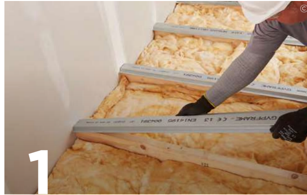
1 Locate Gypframe SIF Floor Channels centrally over the joists.
