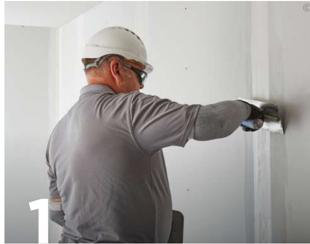
1 Gyproc Joint Tape is bedded into the appropriate Gyproc jointing compound to all board joints and internal corners.
