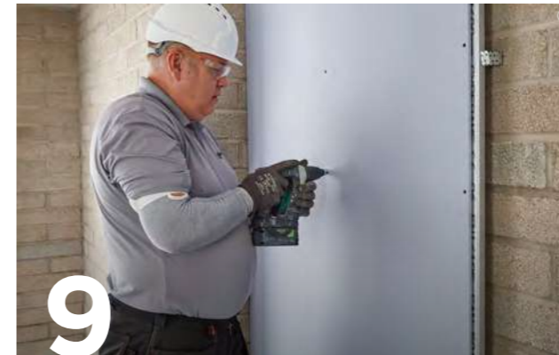
9 Use British Gypsum Drywall Screws to fix Gyproc plasterboards or Gyproc ThermaLine to all framing members.
