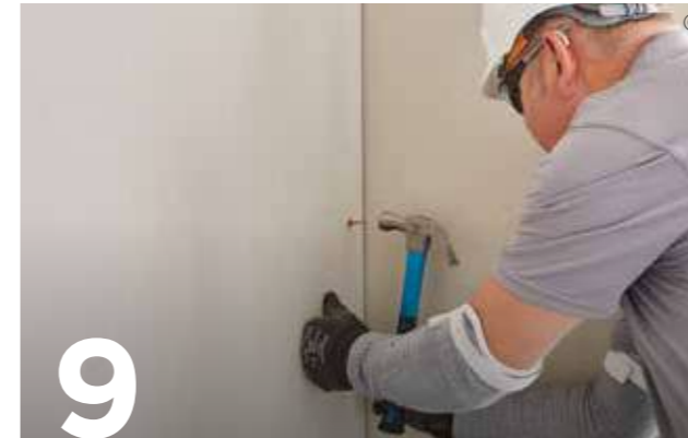
9 When installing Gyproc ThermaLine in this system, insert two British Gypsum Nailable Plugs at mid-height after dabs or blobs have set.
