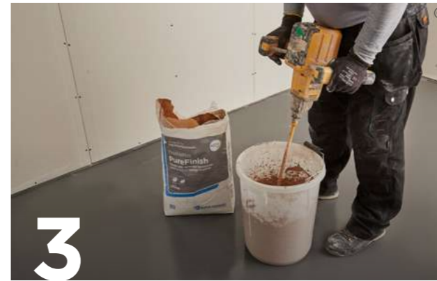
3 Thistle plasters should be mixed by adding to clean water and using clean mixing equipment. Contamination from previous mixes must be avoided as this can adversely affect the setting time and strength.
