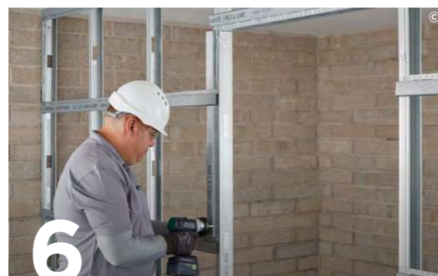
Install Gypframe RB1 Resilient Bars vertically to abutment and door studs to accept perimeter fixings for the Gyproc plasterboard linings.
