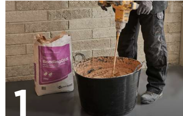
1 Mix Thistle plasters by adding to clean water and using clean mixing equipment. Avoid contamination from previous mixes as this can adversely affect the setting time and strength.
