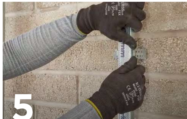
5 Bend the protruding Gypframe Bracket legs back to sit clear of the Gypframe GL1 Lining Channel face. At internal angles position a GL1 Lining Channel is positioned tight into corner, to provide support for the lining.
