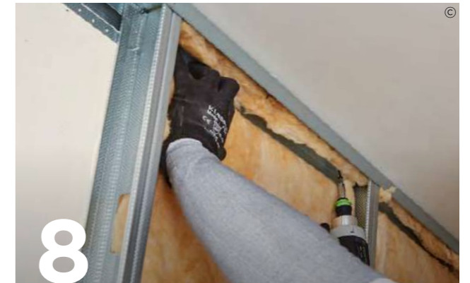
Add Isover Acoustic Partition Roll (APR 1200) insulation to the partition cavity for optimal acoustic performance.
