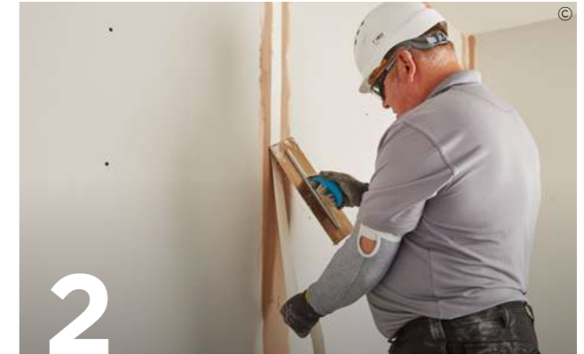
2 Where there is an increased risk of cracking, or where gaps exceed 3mm, the gaps are reinforced with Gyproc Joint Tape bedded in Thistle plaster. In other situations, plasterboard joints can be reinforced with Thistle ProTape FT50 or FT100 glass fibre mesh tape.
