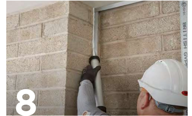
8 Use Gyproc Sealant to seal the perimeter of the lining.
