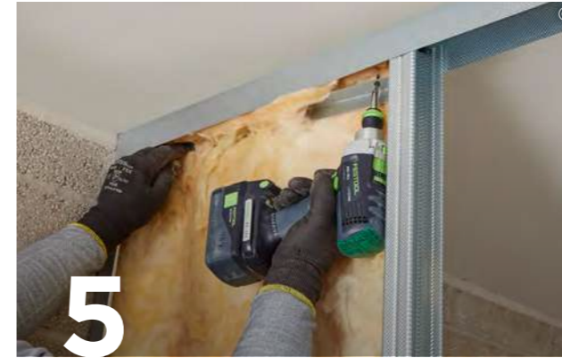
5 Add appropriate Isover insulation (Acoustic Partition Roll (1200) as shown) within the partition cavity to contribute to acoustic and thermal performance where required.
