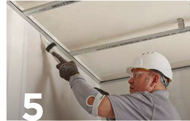
5 Use Gyproc Sealant to seal the perimeter of each frame.
