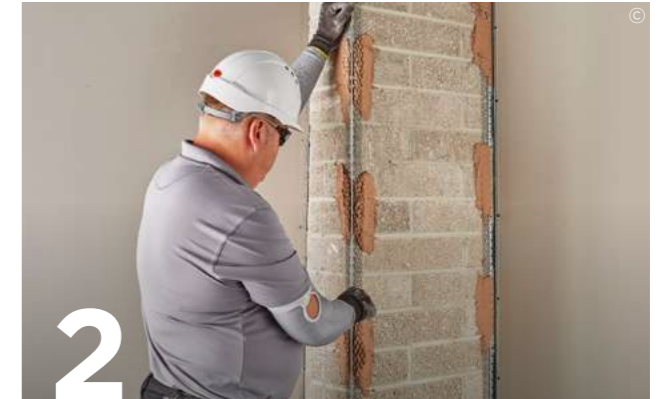
2 Fix a Thistle Plaster Angle Bead or Thistle Plaster Stop Bead to the background by embedding in the undercoat plaster. Where Thistle BondingCoat undercoat plaster is to be applied to plasterboard, reinforce the board joints with Gyproc Joint Tape bedded in Thistle plaster.
