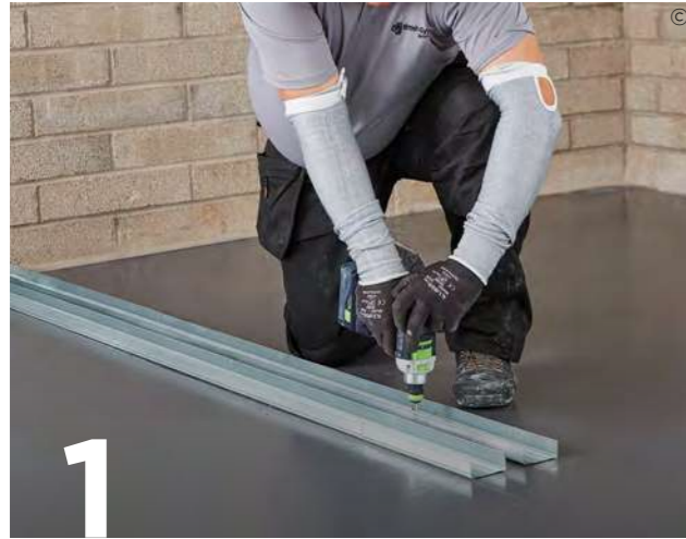
1 Suitably fix the appropriate Gypframe Floor & Ceiling Channels in two rows at the required centres to the floor and soffit.
