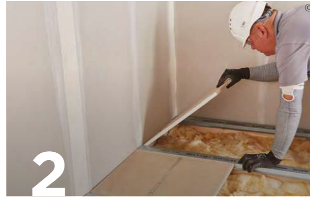
2 Cut Gyproc Plank and position between the channels.
