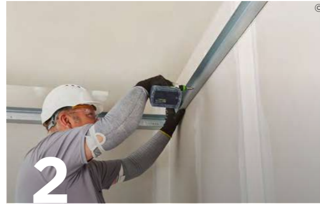
2 Position the appropriate Gypframe Starter Channels within the chosen floor and ceiling channel. Suitably fix to the perimeter at the required centres.
