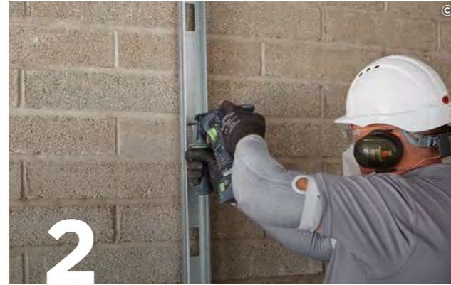
2 Fix Gypframe 'C' studs at appropriate centres to the perimeter construction.
