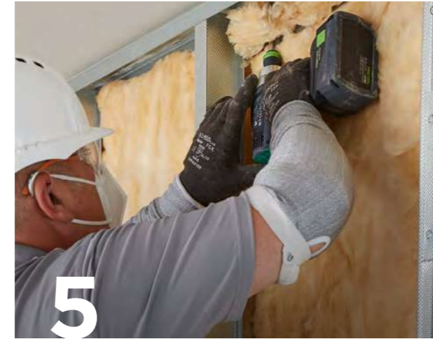
5 Add Isover Acoustic Partition Roll (APR 1200) insulation to the partition cavity for optimal acoustic and thermal performance.
