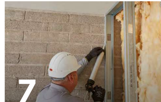
7 Use Gyproc Sealant to seal the perimeter of the partition.
