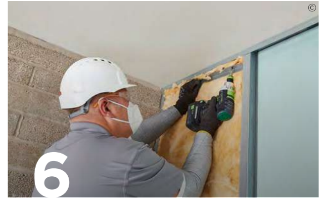
6 Add Isover Acoustic Partition Roll (APR 1200) insulation to the partition cavity for optimal acoustic and thermal performance.
