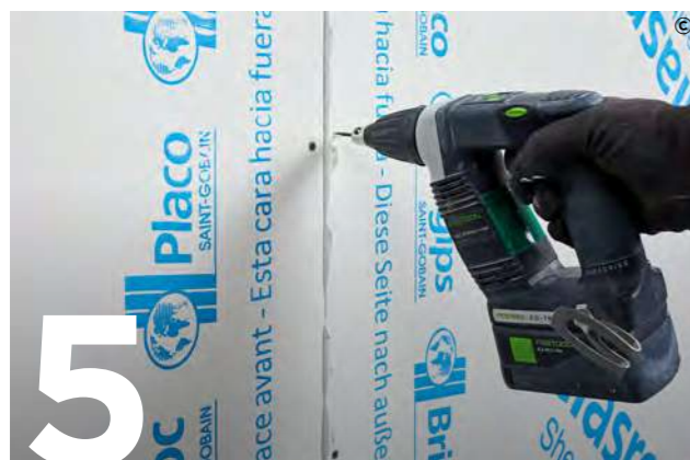
5 Abut subsequent sheets of Glasroc X Sheathing Board up to the previous one ensuring the sealant "mushrooms" out onto the face of the board, fully sealing the joint.
