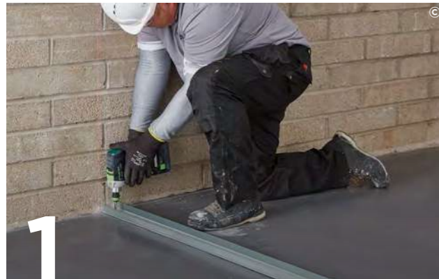
Suitably fix the appropriate Gypframe Floor & Ceiling Channels to the floor and soffit at the required centres.
