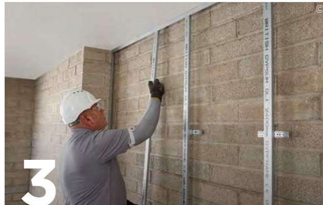
3 Friction fit Gypframe GL1 Lining Channels into the Gypframe GL8 track top and bottom.
