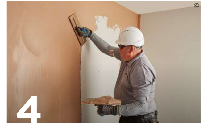
4 Thistle plaster is applied with firm pressure, built out to the required thickness in two applications and trowelled to a smooth matt finish. When applying ThistlePro FastSet Finish, a single mix for both first and second coat is recommended.
