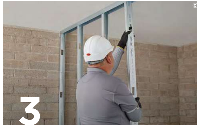
3 Depending on the system, friction fit either Gypframe 'C', 'I' or AcouStuds into the Gypframe Floor & Ceiling Channels at required centres.
