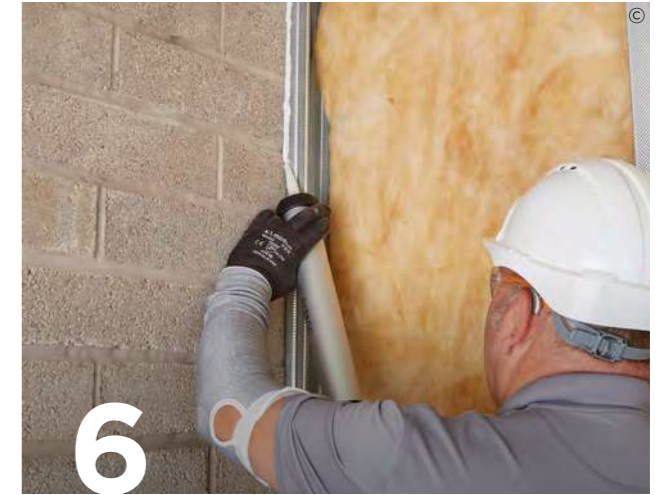
6 Use Gyproc Sealant to seal the perimeter of the partition.
