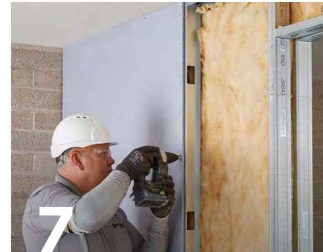
7 Use British Gypsum Drywall Screws and British Gypsum Jack-Point Screws to fix Gyproc plasterboards to the Gypframe framework.
