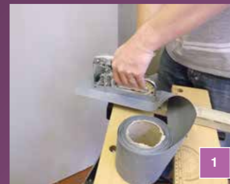
25 x 50mm treated timber battens should be used to install Eco-Liner. 100mm DPC strips should be cut and stapled to the back of the battens prior to fixing to the wall. Mark the walls to indicate the position of the battens.
