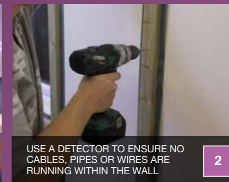
Fix vertical battens to the wall at a maximum of 600mm centres. Hold timber in place, drill through the timber into the wall and secure in place using wood screws and wall plugs or nailable plugs (see fixings). Timbers can be packed out to ensure a level surface. Horizontal battens should be installed at the top and bottom of the wall.
