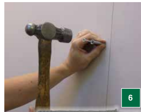
When fully dried (at least 24 hours), drill through into the masonry and fix a minimum of 2 nailable plugs per board, 15mm in from each edge (approx. 1600mm up from the floor). Plugs should penetrate a minimum of 25mm into the existing solid masonry. Tighten the screw heads to just below flush.
