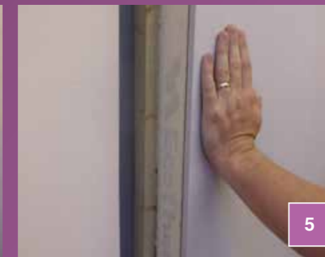
Place Eco-Liner in position. The board must meet the centre lines of the timber battens. Board joints must be staggered (break bonded).
