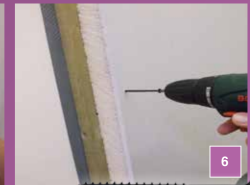
Secure Eco-Liner to the timber battens using drywall screws at 300mm centres and 200mm centres, around openings / external corners. The fixing should penetrate at least 25mm into the timber. Fixing should be no less than 10mm in from the edge of the board.
