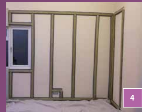
Fix battens around all wall edges, openings and services. Come round the internal wall a minimum of 400mm.
