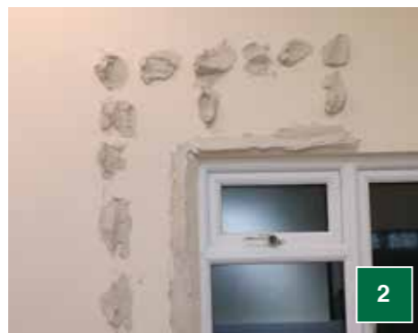
Trowel a continuous ribbon of adhesive around all wall edges, openings and service penetrations.
