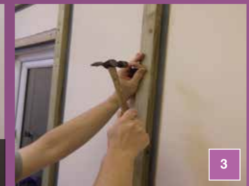
Fixings should penetrate a minimum of 45mm into the existing solid masonry and fixings should be no more than 600mm apart and 75mm in from the end of each timber batten.
