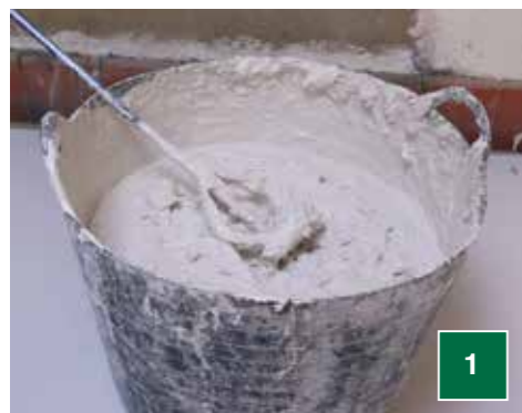
Mix up drywall adhesive as per manufacturer guidelines.
