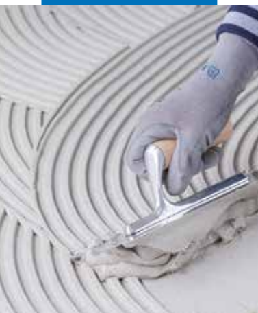
Spreading Adesilex P9 white
