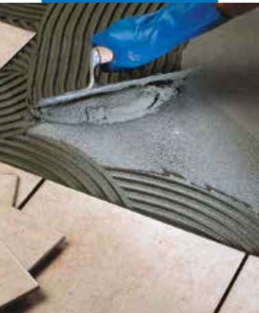
Installation of single-fired tile on floor
