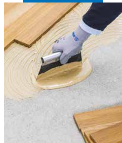
Spreading the adhesive
