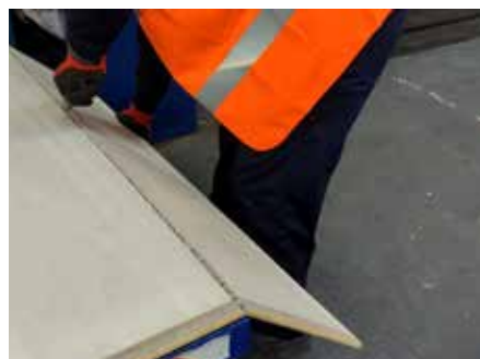
Score and snap method for cutting
