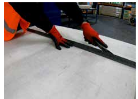
Score and snap method for cutting
