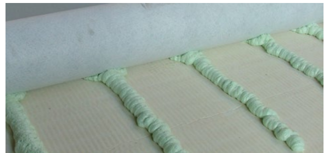
A bonded membrane incorporating HardRock Multi-Fix (DD)
