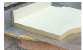
Typical Installation - Timber Deck
