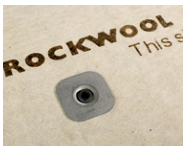
Installed plastic tube and washer
